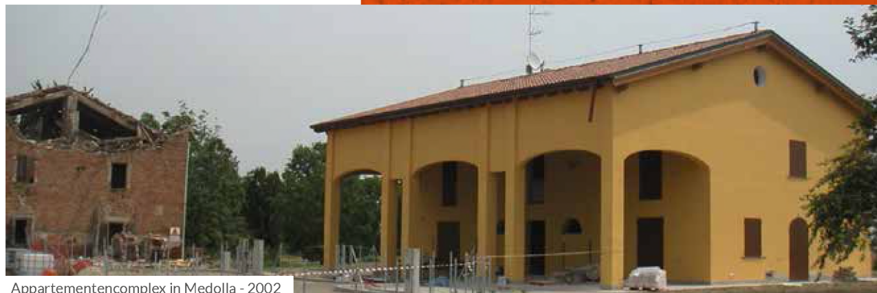
Appartementencomplex in Medolla - 2002
